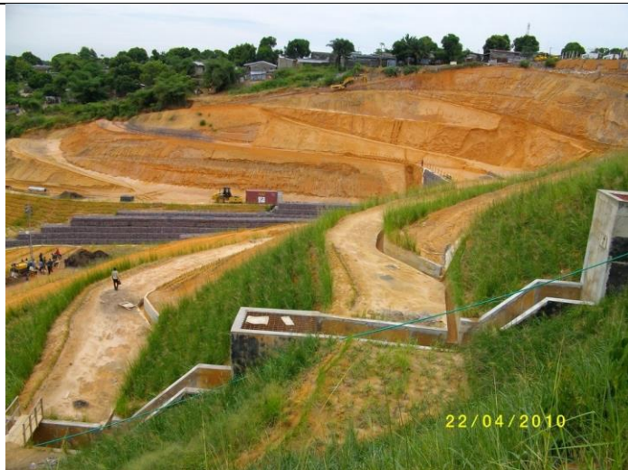
1. Other side of Casis erosion site while planting vetiver
