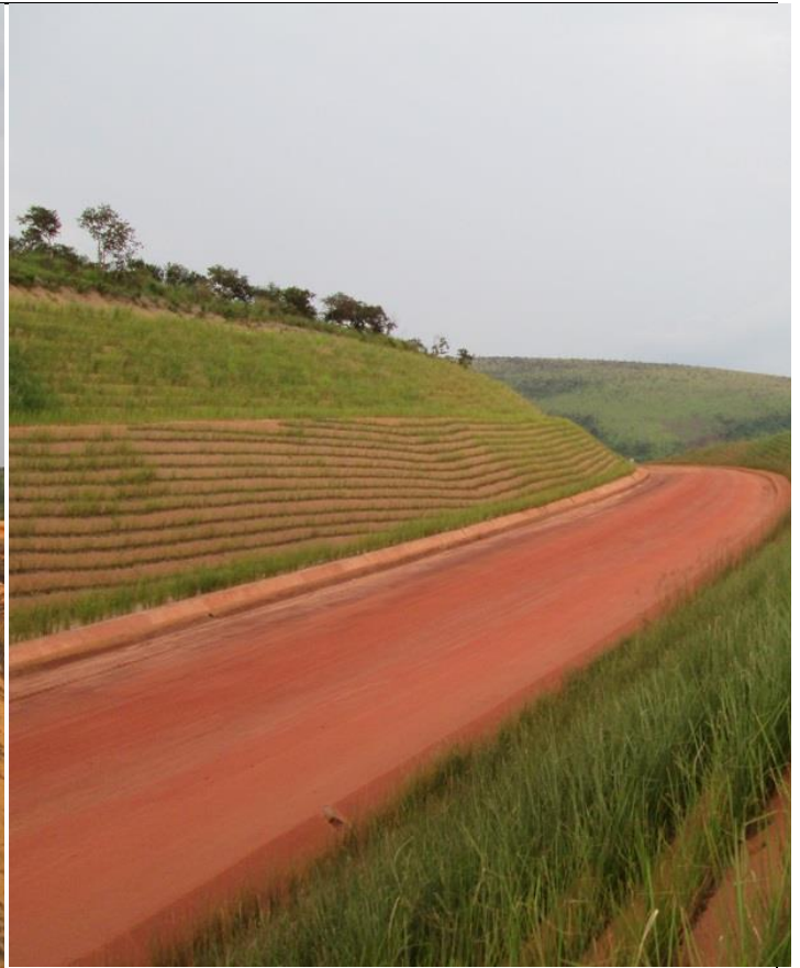
Road slope totally protected by vetiver grass, some months later
