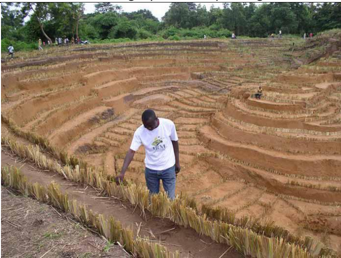
4. site checking after vetiver planting
