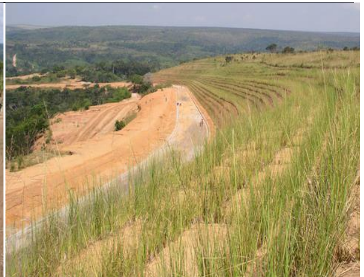
2. Road cut embankment totally stabilized some months after vetiver planting
