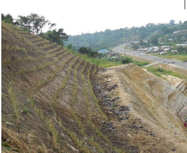
On going vetiver plantation on steep slope in Uganda republic , august 2013
