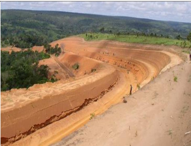
1. Road cut embankment before vetiver planting may 2007
