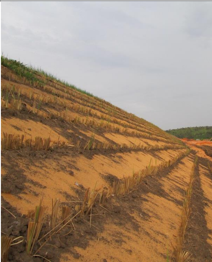
Vetiver plantation on steep slope of road, November 2013
