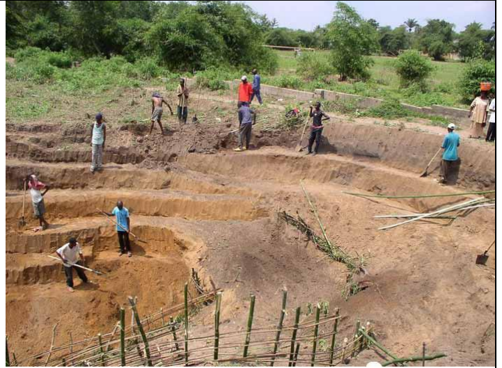
2. gully site reshaping before planting vetiver at Kikwit
