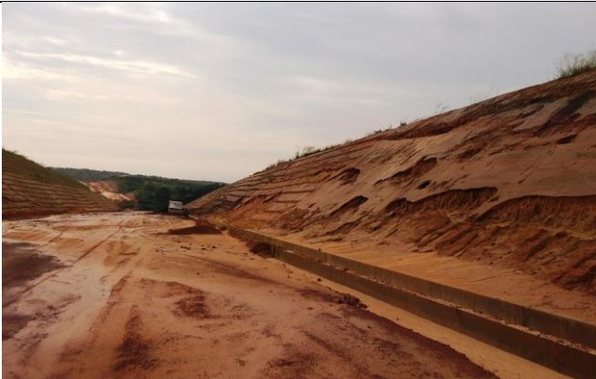
Vetiver plantation on steep slope of road, November 2013
