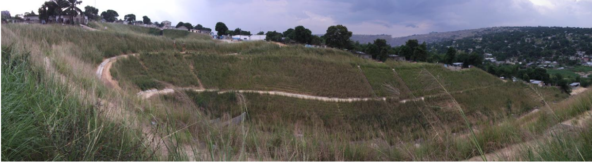
2. Same site totally stabilized, may 2014
