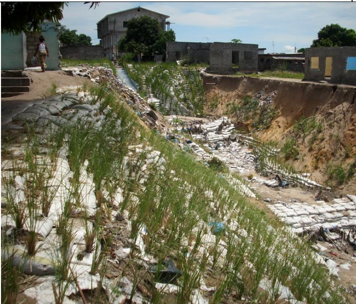
3. The progress of work at Boukeni site, one month later
